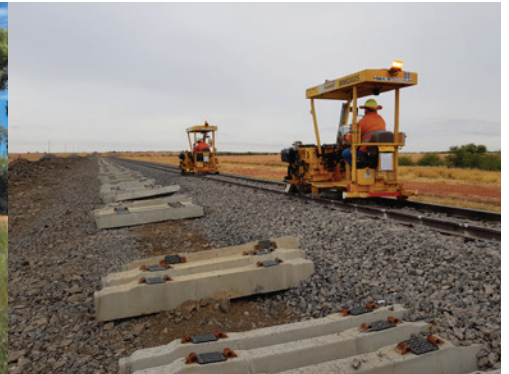
QR's re-sleepering work between Richmond and Hughenden in May
